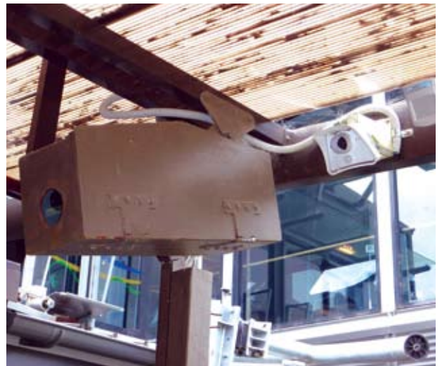
A compact Robotix megapixel camera beside one of Scenic World's original CCTV housings
